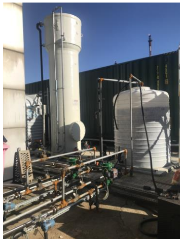
GRANULAR BIOLOGICAL REACTOR (AIRLIFT)
