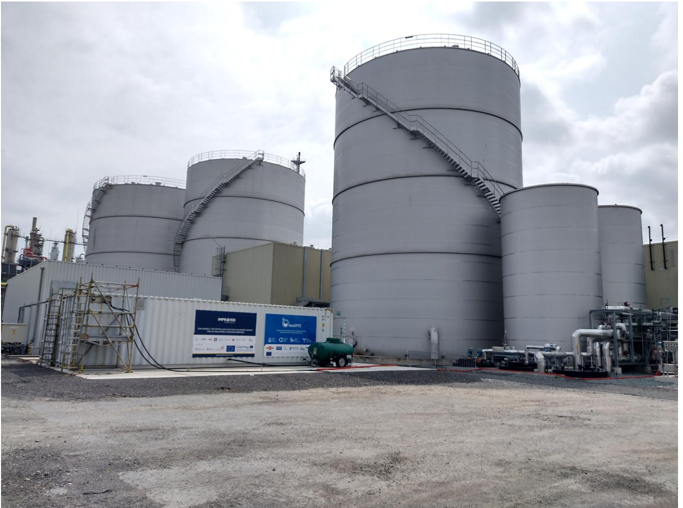
The Improved containers on site at BASF Antwerp
